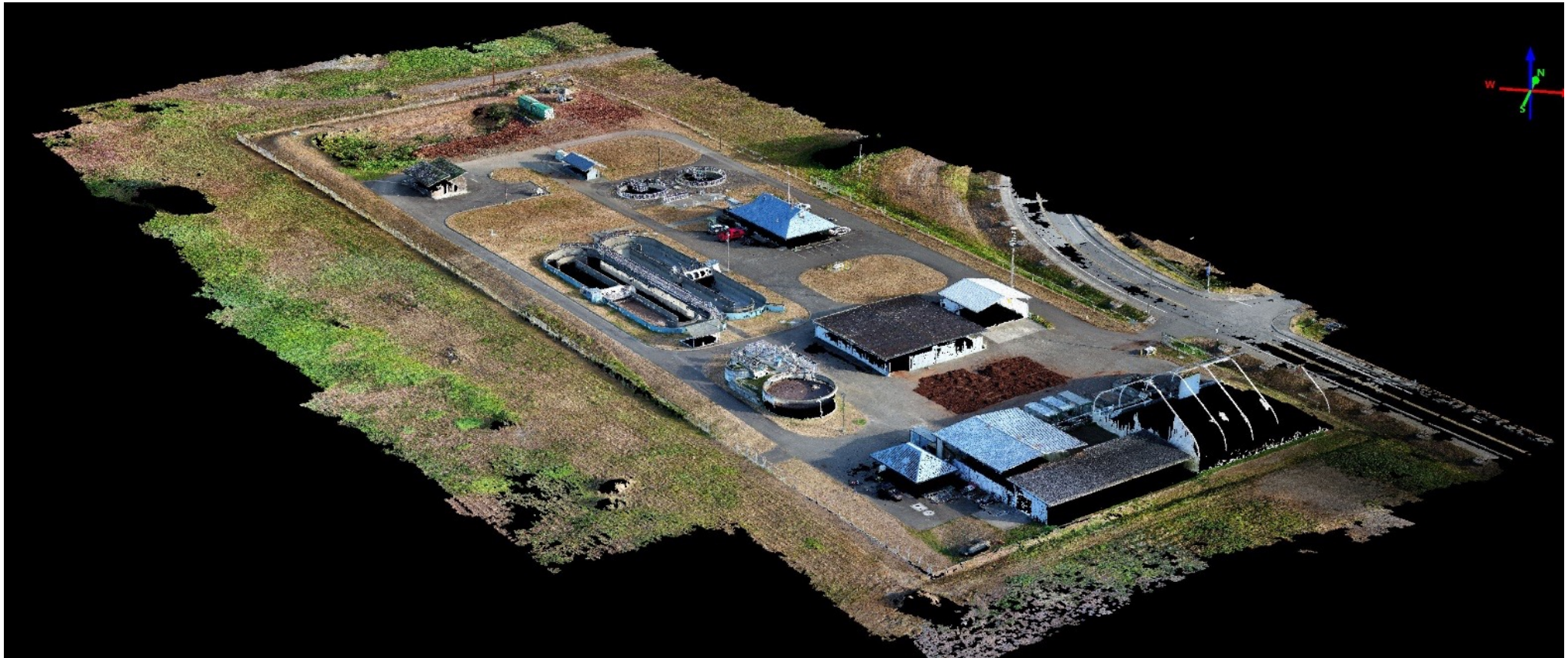
Wastewater Treatment Plant
