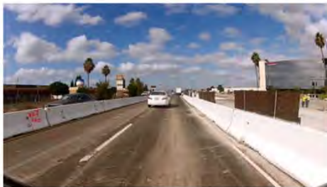
Exhibit 10-16 Example of Minimum Lateral Clearance in Work Zone
